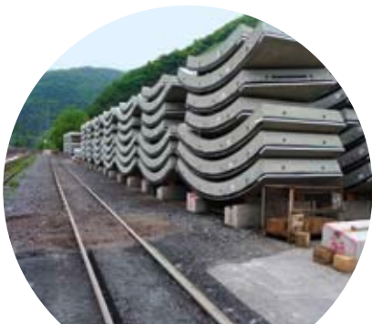
TUBBING The curvature of the precast concrete parts used for lining the freshly bored tunnel section is clear to see.
