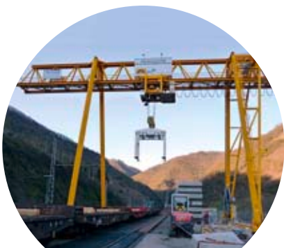
INTERIM STORAGE The precast concrete parts are produced by Max Bögl and delivered by DB Schenker Rail to the site on the Moselle river.
